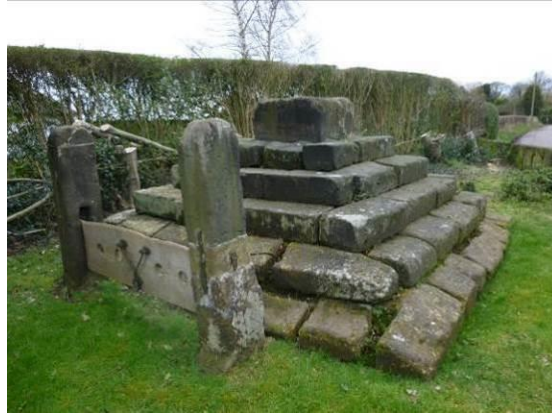
Dislodged steps to cross base and cracks to stocks
