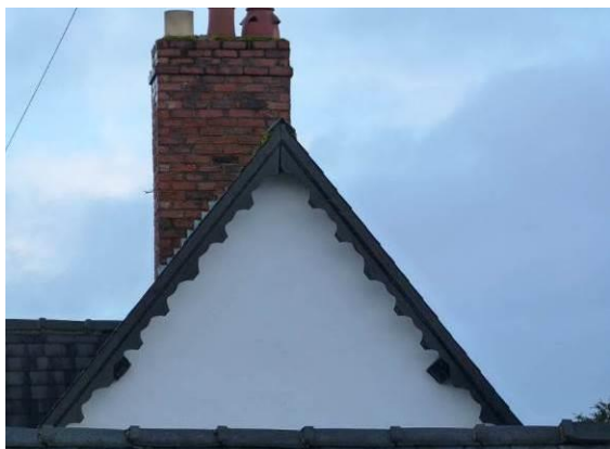
Detail of later applied barge boarding
